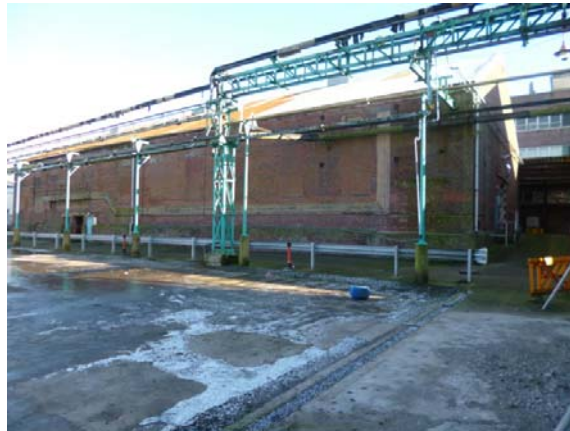
Figure 4 TCP Warehouse Building
