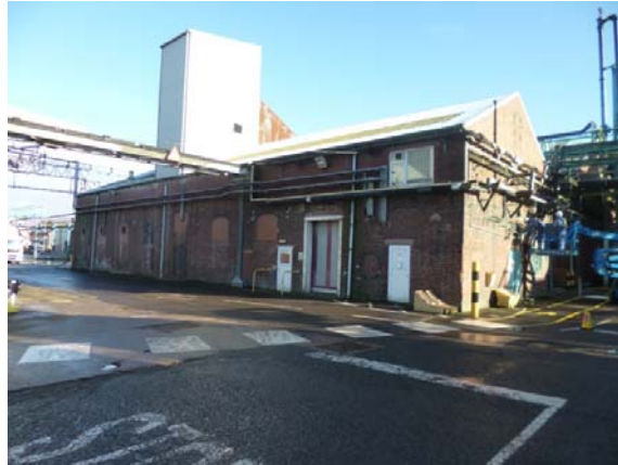
Figure 3 TCP Plant Building
