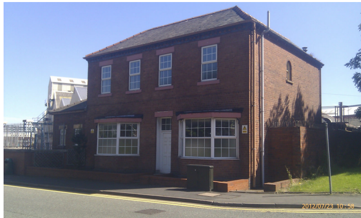
Figure 1 Location of New Boundary Wall when Building is Demolished.
